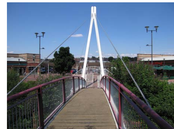
Footbridge: Vue complex to Armley Mills
