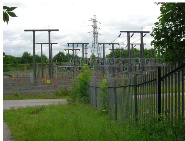
Electricity switching station
