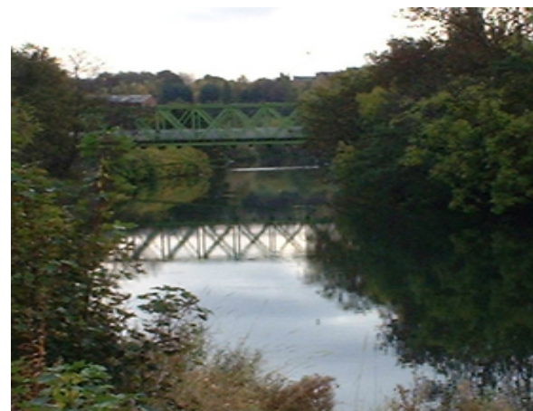
River Aire: Redcote Bridge
