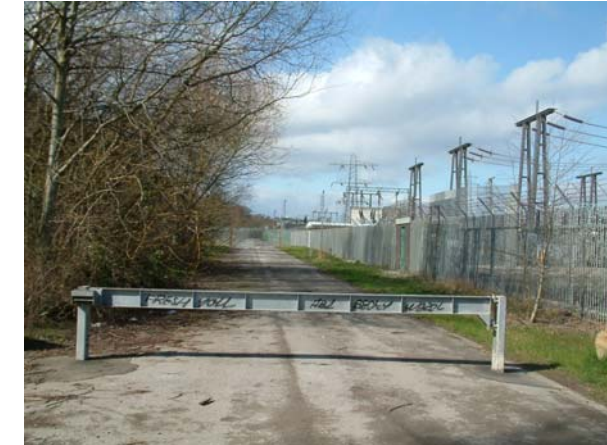
Existing track by switching station
