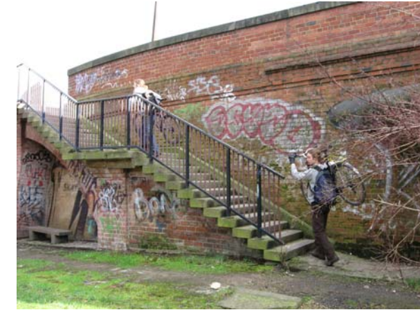
Poor connections to Canal towpath
