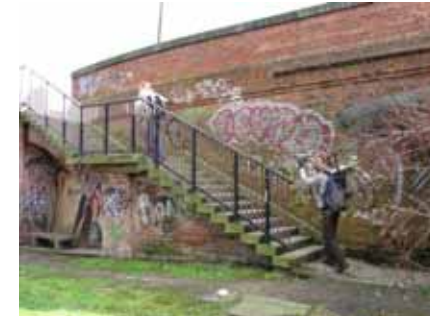
Poor connections to Canal towpath
