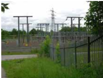
Electricity switching station
