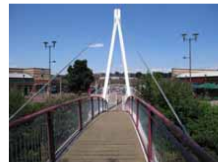
Footbridge: Vue complex to Armley Mills
