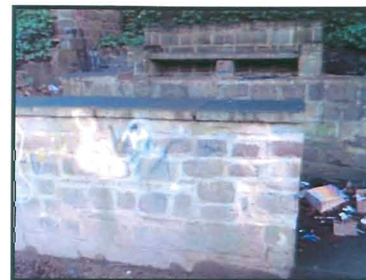
Signs of vandalism Goitside Walk
