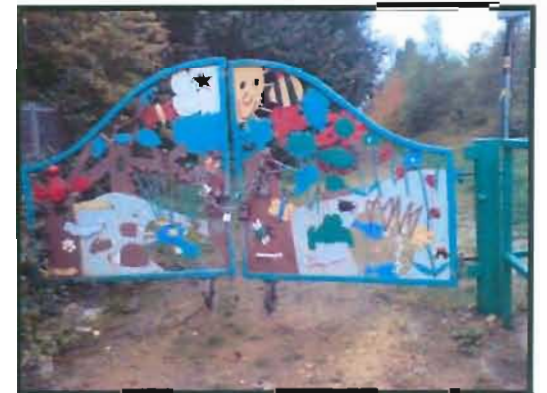
Existing gates and barrier system restrict access to both cyclists and disabled users
