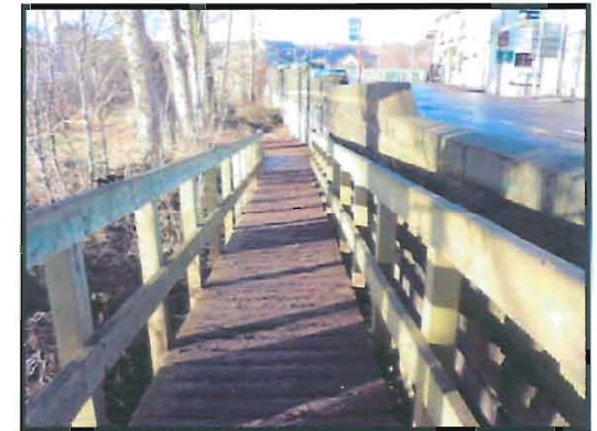
Existing ramp entrance at Bridge Road
