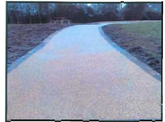
Bituminous base course with sprayed gravel surface
