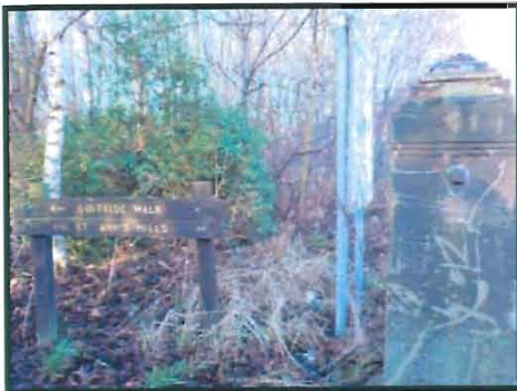
Existing signage in disrepair
