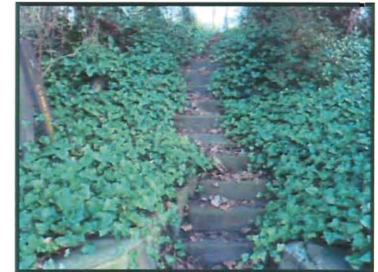
St Ann's Mills pedestrian entrance
